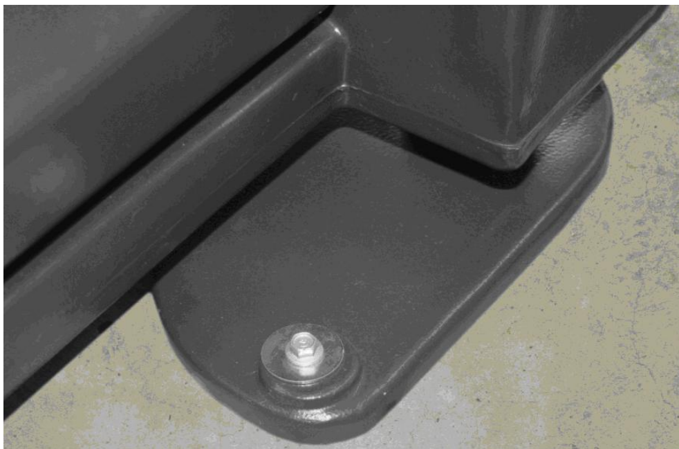
Figure 7. Fixing to pad.
