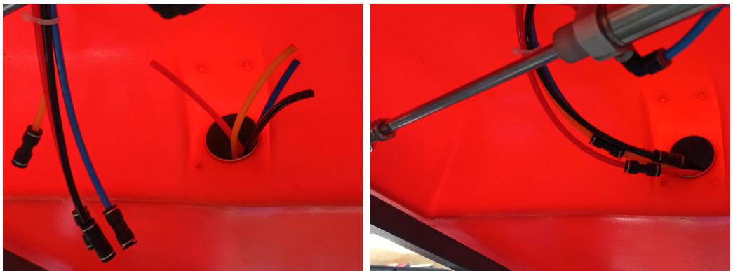
Figure 18. Attaching air lines.
